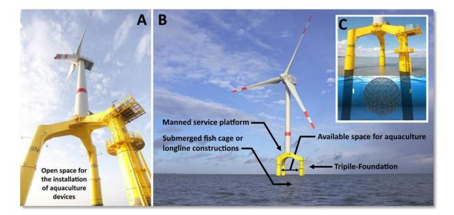
Figure 7 – Tripile foundation for the secondary use for fish cages. (A) shows the open space within a tripile foundation to be used for aquaculture purposes, (B) displays a lateral view of the Bard-Wind turbine and the access to the fish cage, and (C) is a edited photo to give an idea how a fish farm, such as an Aquapod, could be moored below (Buck & Krause 2012).
