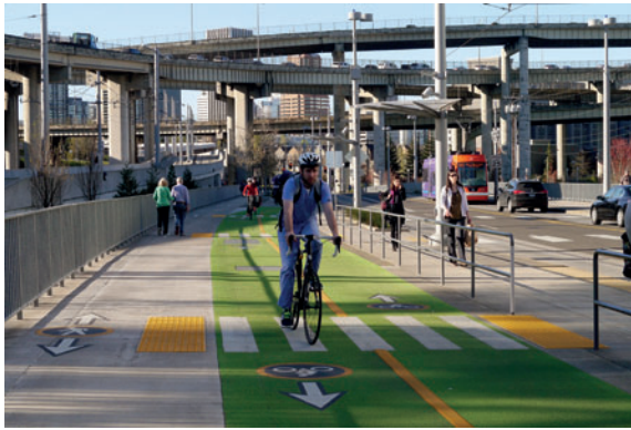
Figure 2.4-6 Breaking up the path dependencies of a car-oriented city. Portland, USA. Source: Mareike Kroll/WBGU
