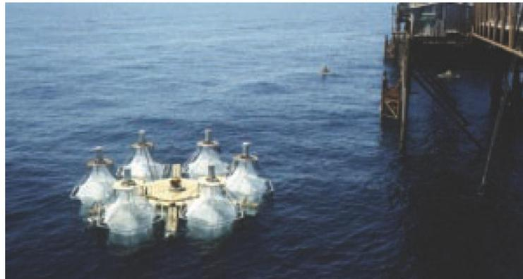
Figure 1 – Submersible cage complex «Sadco-Kitezh» (consisting of 6 individual cage modules) disposed near an offshore oil-rig in the Caspian Sea in 1988 (Burgov 2006).
